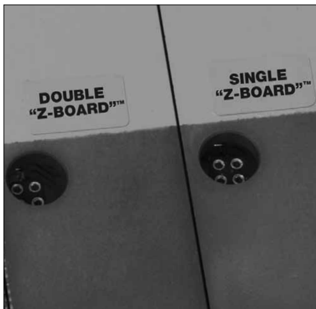
Label on manifold block indicates Installed "Z-Board"™ type.
